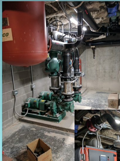
Above: Circulating Pumps Right: Boilers
