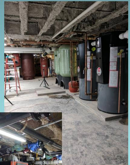
Above: Water Softeners and Heaters
